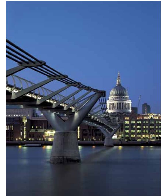
Figure 1. View of the Millennium Bridge over the Thames in London. Photo ©Nigel Young/Foster + Partners.
