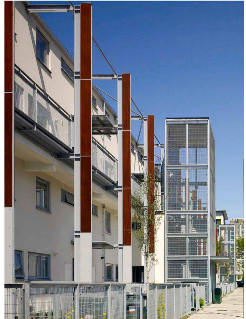
Figure 3. Brook's Road: Part of the completed project. Photo ©Bell Phillips
