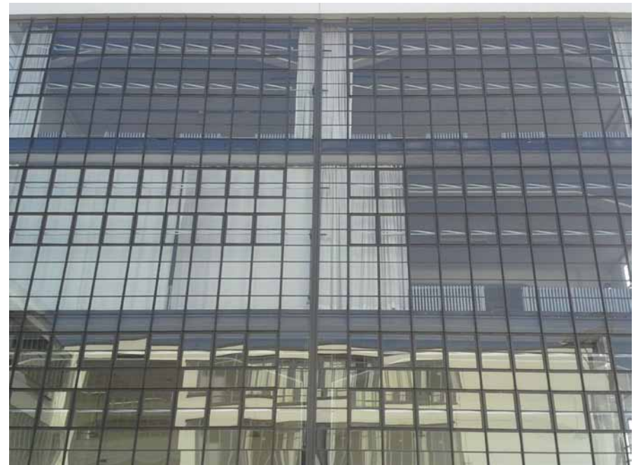
Figure 7 Glass facade for building including classrooms and labs at the Bauhaus school in Dessau, built in 1933. Photo by Magnus Rönn, 2010.
