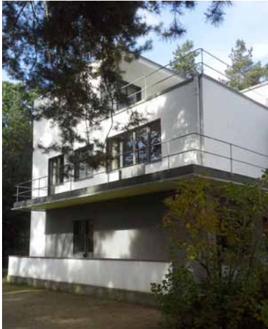
Figure 5 Restored houses for the dean at the Bauhaus school in Dessau, originally built in 1933 and damaged by the Second World War. Photo: Magnus Rönn, 2010.
