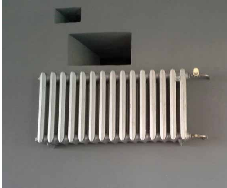
Figure 9. Wall mounted radiator 1933 at Bauhaus school in Dessau. Photo by Magnus Rönn,
