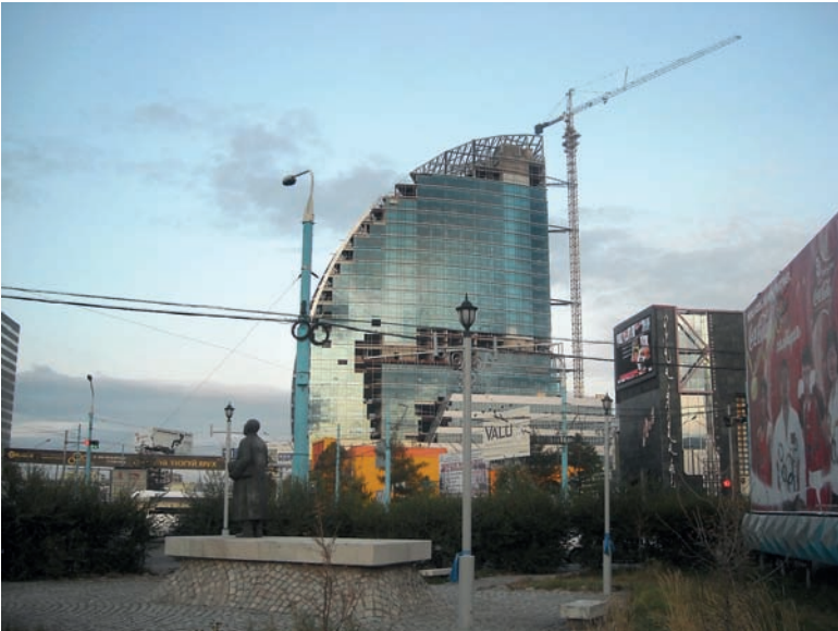
The Pregnant Lady or the Blue Building under construction in Central Ulaanbaatar in 2008, with the statue of Zorig, a hero of the Democratic Revolution of 1990, in the foreground. Zorig's murder in 1998 still remains unsolved.
