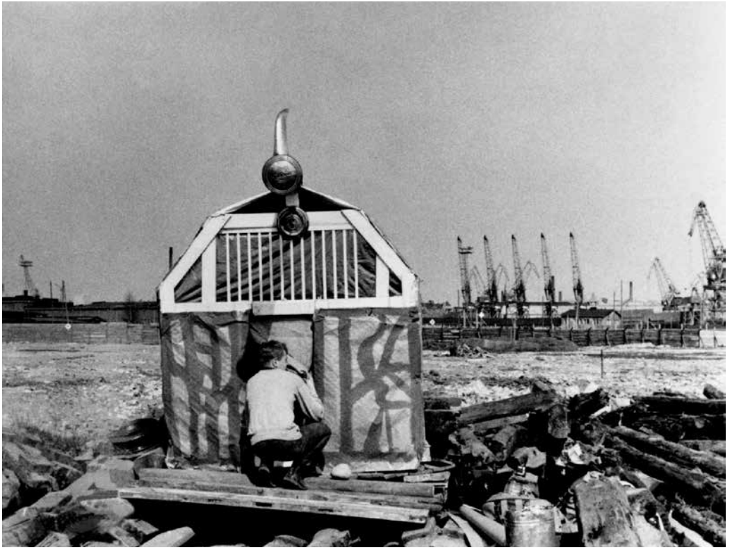
FIGURE 1.3. A temporary shack built by students in Jätkäsaari, Helsinki. 1966. Photographer unknown (possibly Kaj Franck). Design Museum, Kaj Franck Archive.
